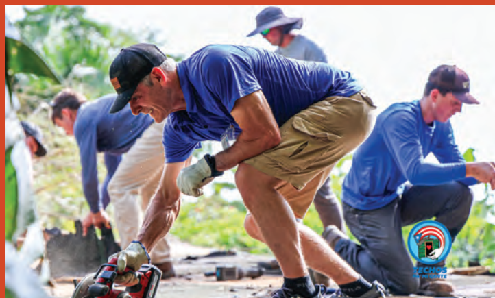
Volunteers participate in repairing 70-year-old Hilda's roof.
