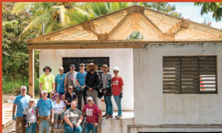
Volunteers sit for a group photo while completing repairs on Jose's family home.
